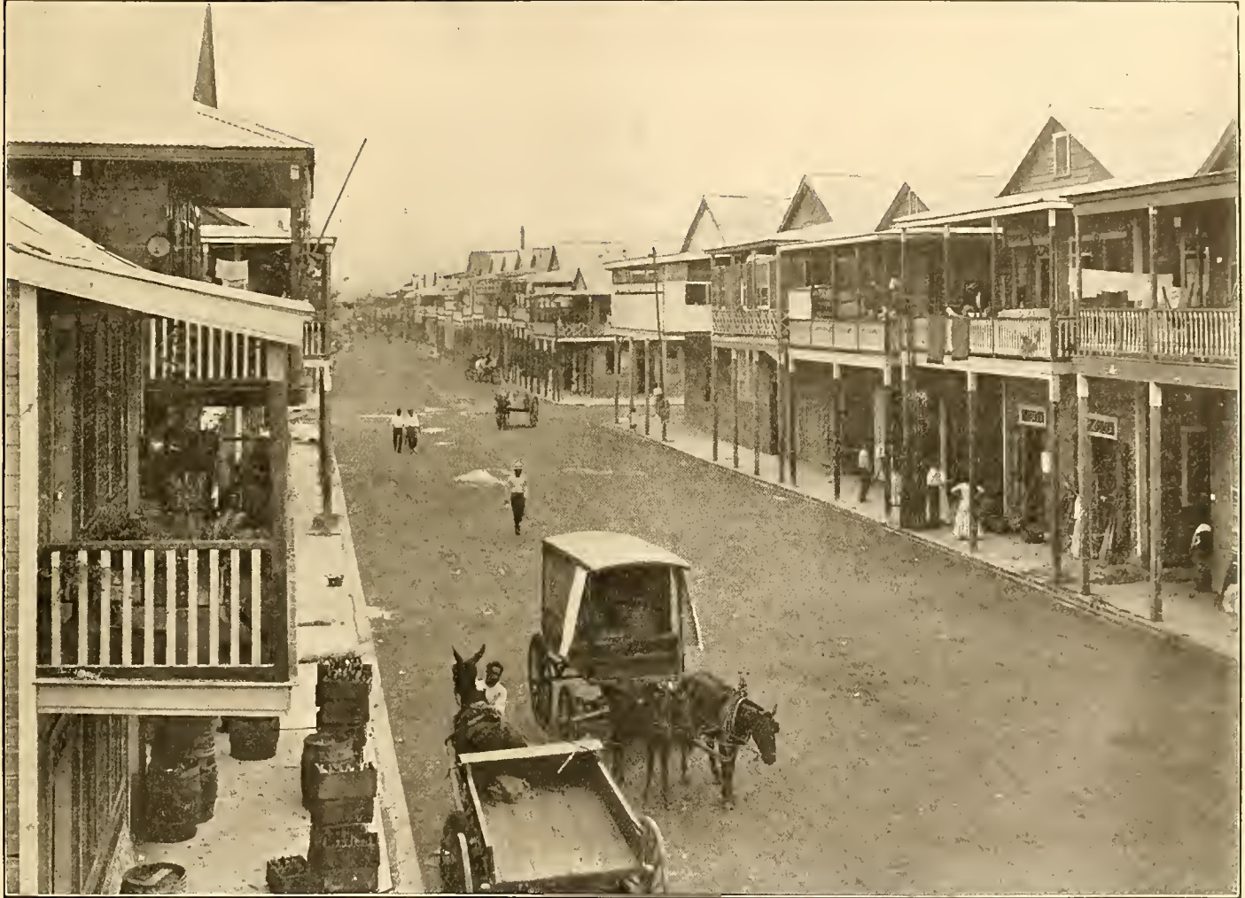
D STREET, COLON, PAVED
